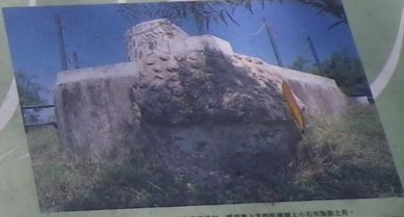
砲台位於海濱的砲兵觀察所，入口及觀望口已封，唯望上方的砲台上小石作偽裝之用。The observation post located at the end of Hardsch Road, its entrance and viewing slits have been sealed. There were lumps of cement pasted at the upper part of the viewing slits presumably for camouflage.
